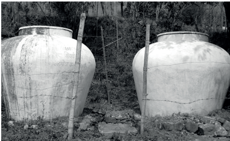
Figure 3.4 Two 3,000 liter Thai jar storage tanks
