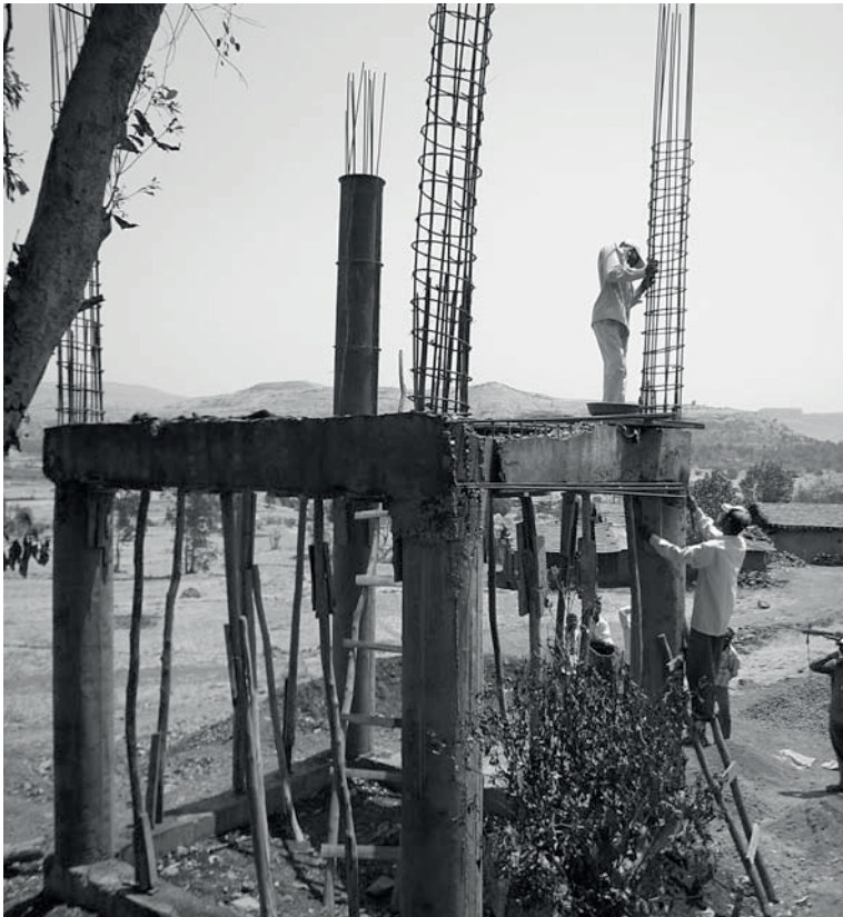
Figure 11.6 Construction of the 26,000 liter overhead tank
