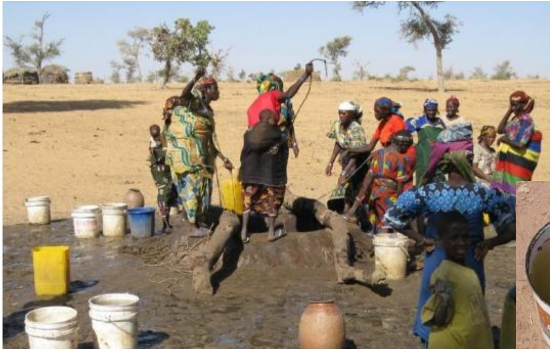
Ropes drag in the mud, carrying dirt and disease into this Matameye department traditional drinking water well.
