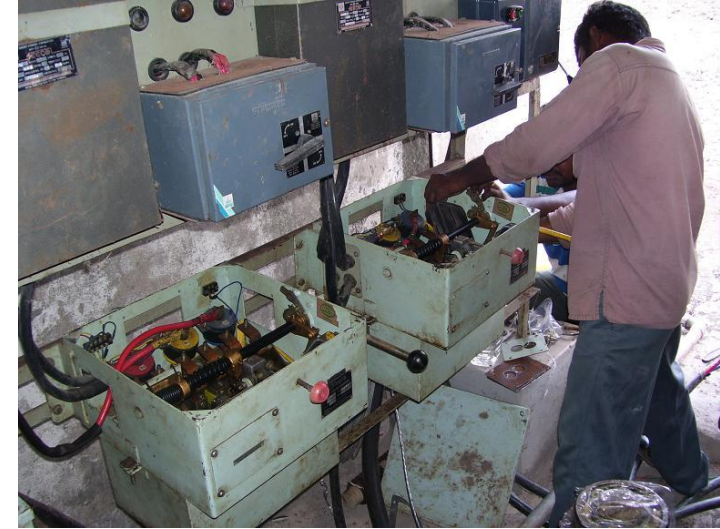
Repairs to Panel Board
