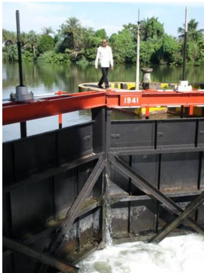
Plate 17 Locks along the Main Canal of KWD
