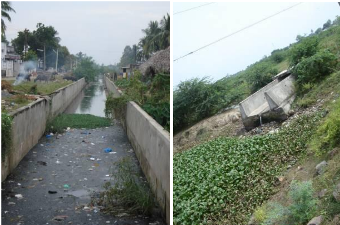
Plate 11: Open drain and its outfall outside Bapatla.
