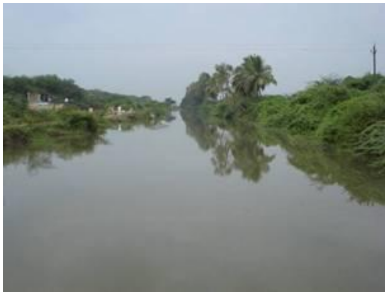
Plate 4: Raw water pumping station alongside branch canal at Bapatla
