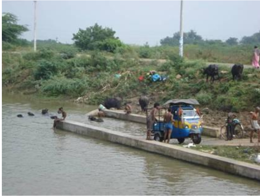
Plate 8: Ramp to facilitate access to canal for all kinds of in-stream uses.
