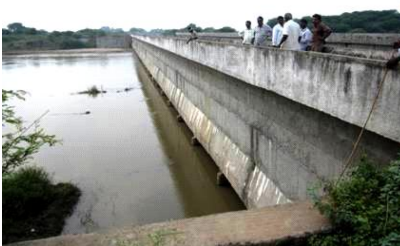
Plate 18 Undertunnel: Commamuru canal crossing the Nallamada drain.
