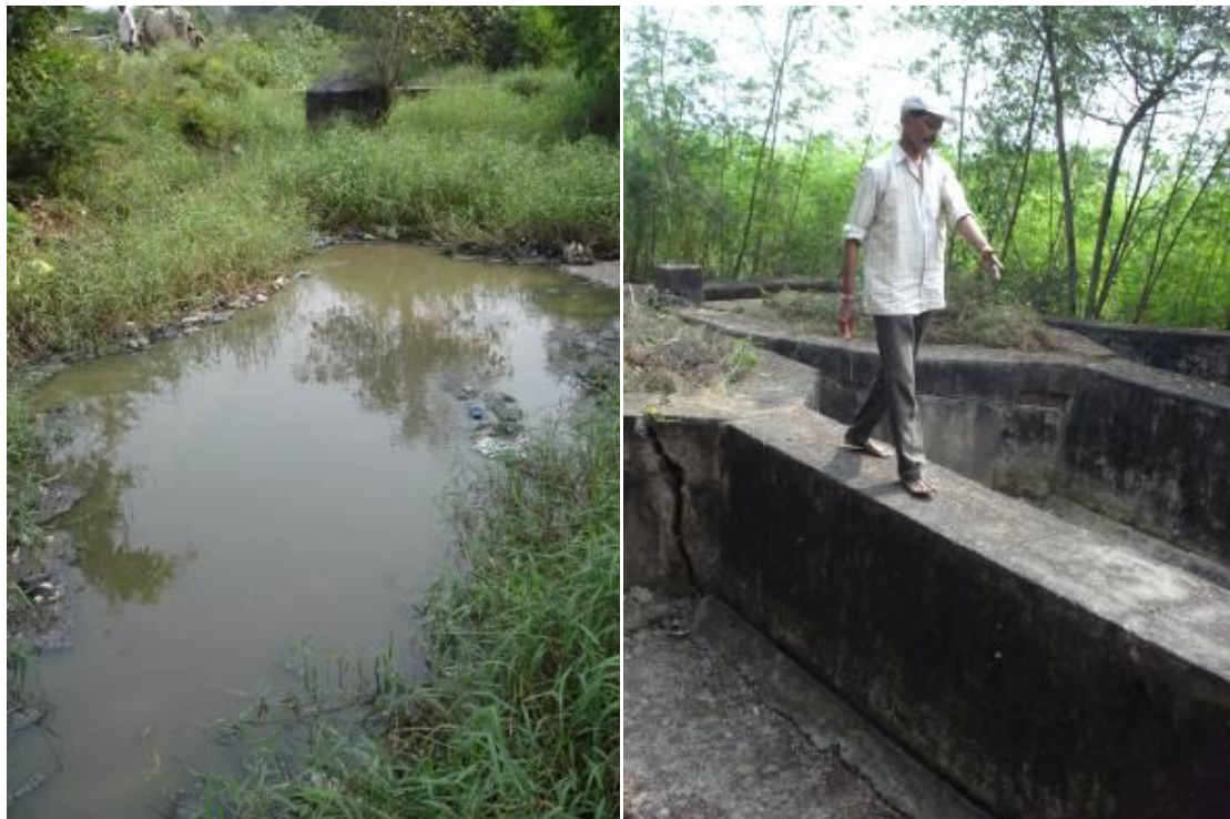
Plate 12: Open drain with sewage and caretaker explaining the abandoned wastewater treatment plan.
