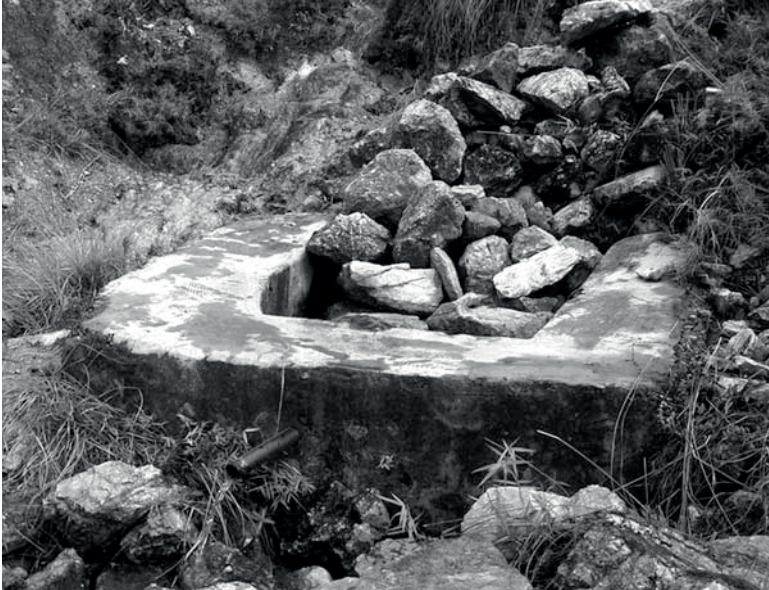
Figure 4.3 Intake from Dhap Pani mul spring
