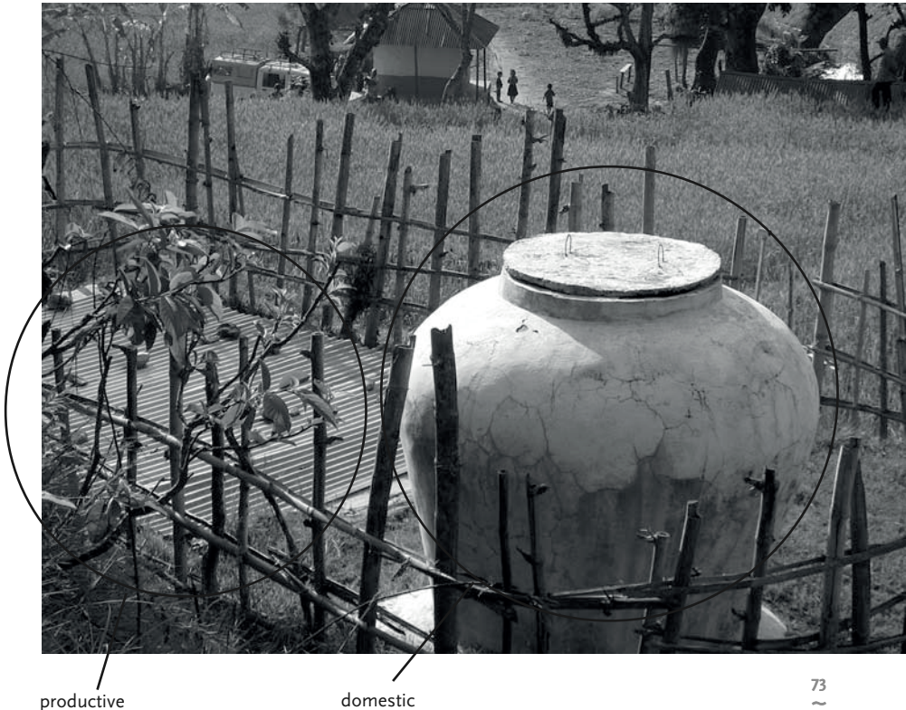
Figure 4.4 Two storage tanks for Senapuk MUS system – domestic with productive overflow
