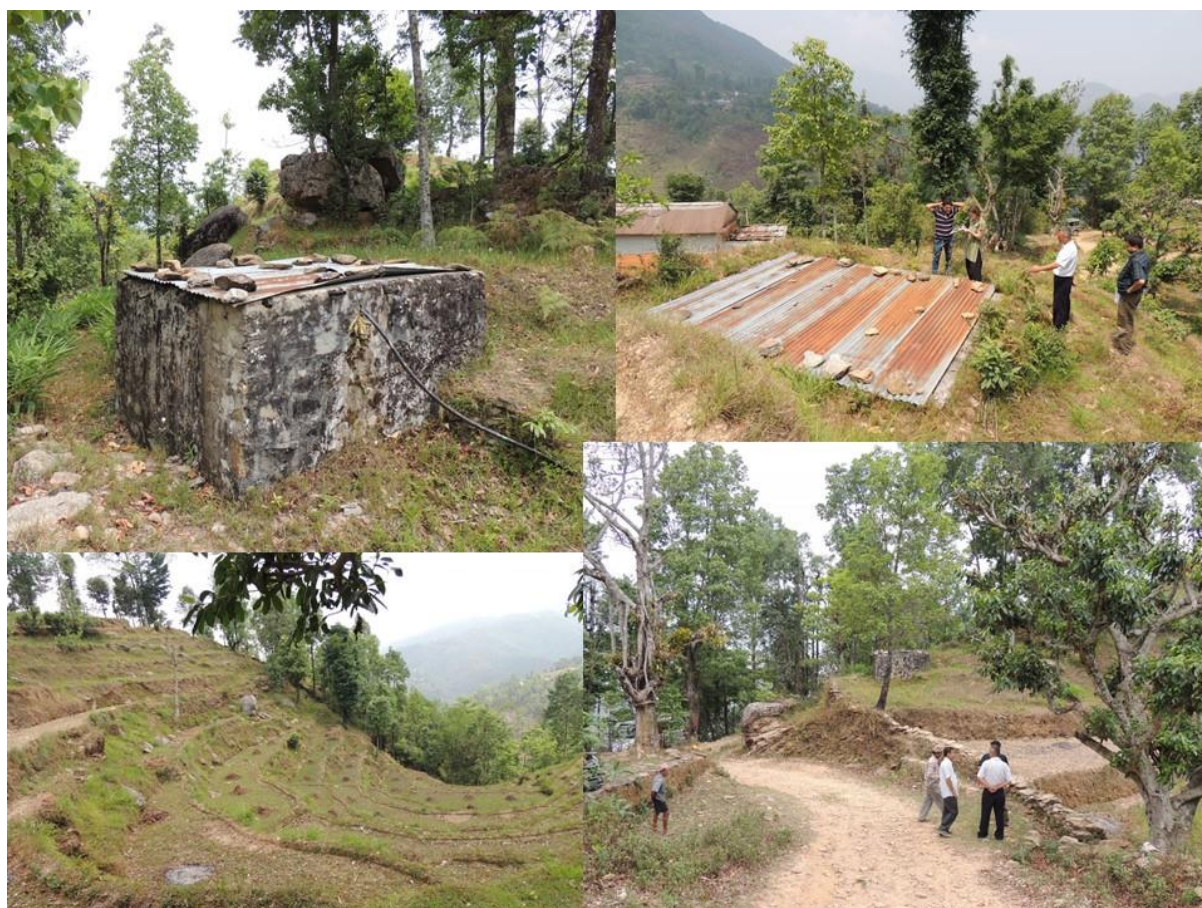
Photography 2. Series of photos from Bhandarekhola: top left: tank built by the government in 1989 for drinking water supply; top right: tank built by the SIMI project in 2004 upstream of the government tank; bottom left: view of the khet land; bottom right: the road which was built in 2007
