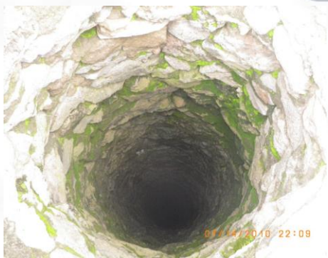
Figure 3. Family well lined with stone masonry.
