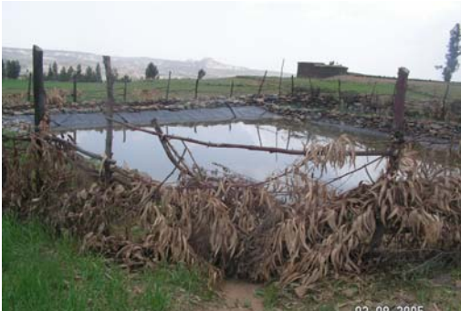
Well fenced plastic lined Trapezoidal pond
