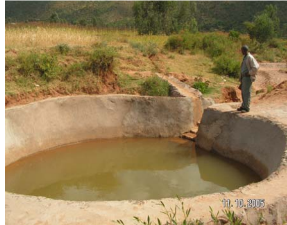
Figure 13. Trapezoidal shaped plastic lined pond with high evaporation surface and Cylindrical shaped pond with low evaporation surface area.
