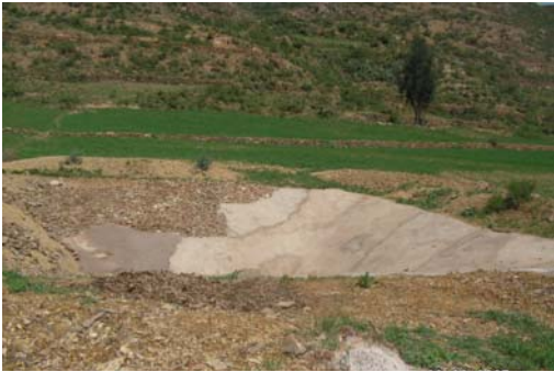
Cement lined Trapezoidal pond
